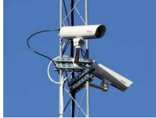
The FLIR A615's high resolution enables Termisk to reduce the number of cameras needed to scan the whole area, which makes it very economical.
