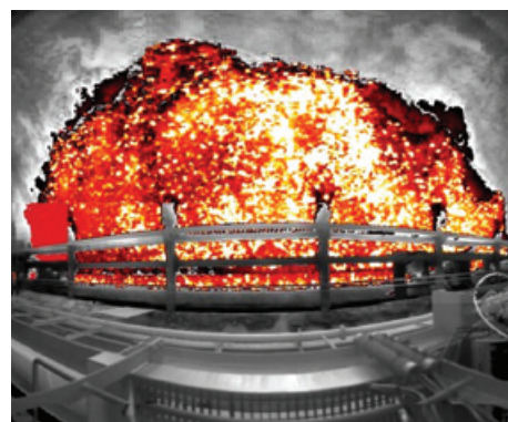
Cokes production: hot areas that have not been cooled down can be identified immediately with the PYROsmart system. In combination with a fire monitor, the parts that are too hot can be cooled immediately.
