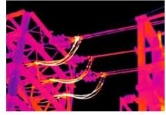
High voltage electrical installations tend to heat up before they fail. By monitoring HV-equipment continuously with thermal imaging cameras costly breakdowns can be avoided.
